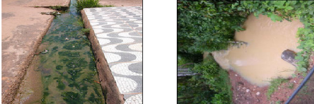
Image 3 - Open air tubulation (left); sewage tabulation loading (right)
